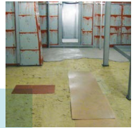
ROCKWOOL A-60 floating floor system (example)
