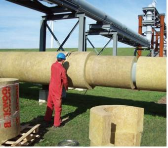
A ROCKWOOL field technician applies ProRox<sup>®</sup> PS 965 with CR-Tech<sup>™</sup> insulation sections in the field. The lightweight, mandrel wound sections apply easily and efficiently, with minimal downtime and safety risks.
